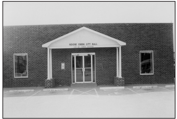
Figure 12: The photograph shows the façade of the third Goose Creek City Hall, after workers installed front windows in 1989.
